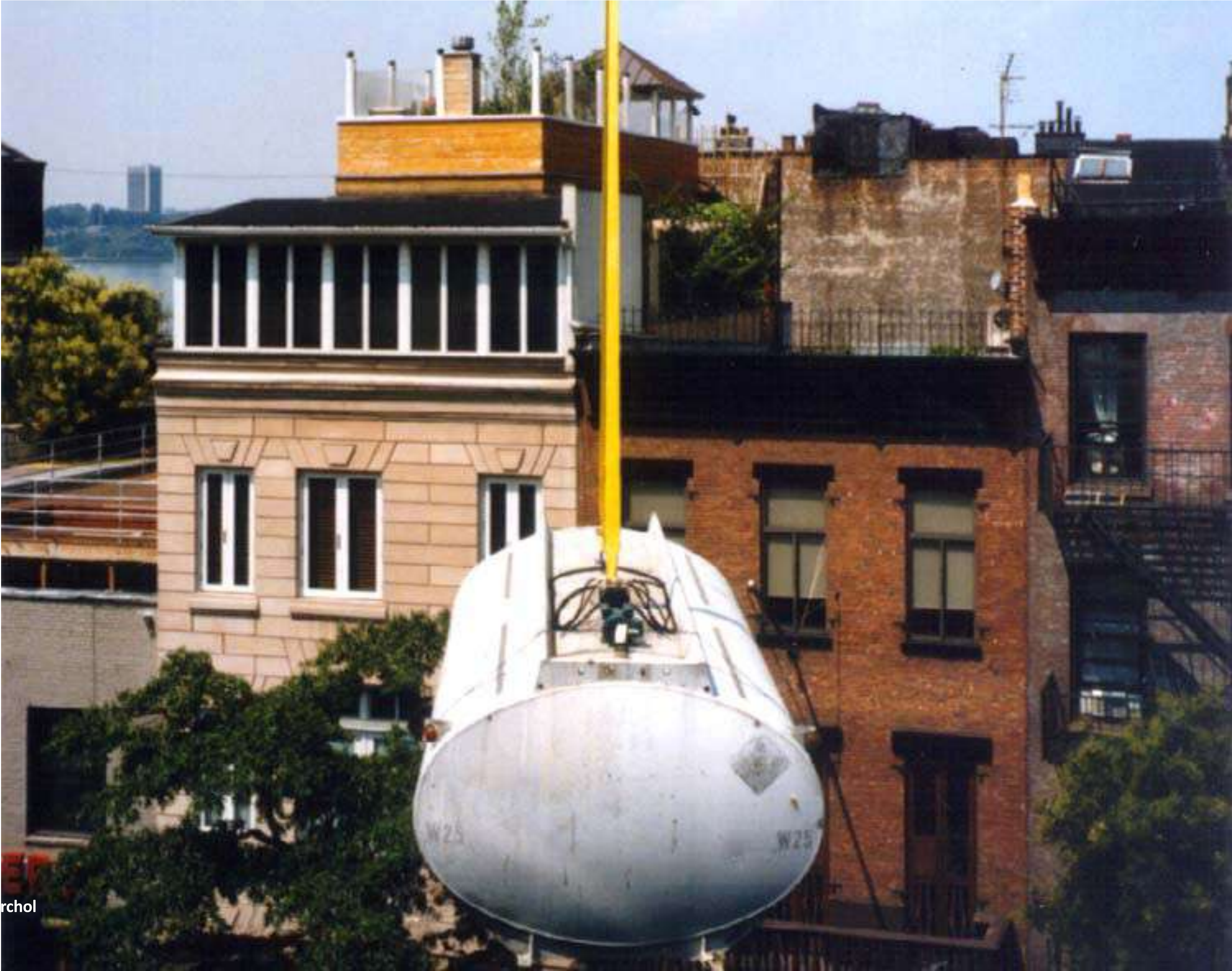
MORTON LOFT 2000 WEST VILLAGE (NY)
